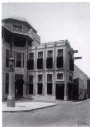
Ills.6 Office building Nillmij, Office building Nillmij, Heerenstraat/ jl. Let. Jen. Suprpto, Semarang. Design: Th. Karsten (1916). People in the Indies spoke of 'grille architecture': concrete grilles provided ventilation which was so necessary. The buildings in Semarang, Djocja and Bandung offer particularly fine examples. Sometimes, as in this building, stained glass designs were mounted in the grilles.
