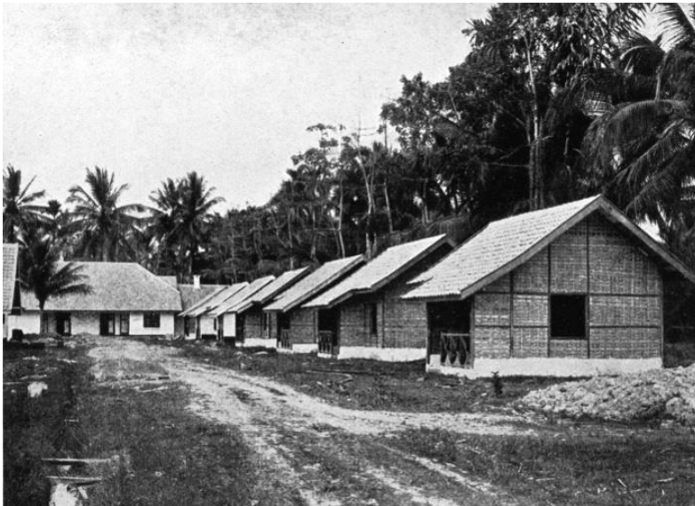
Semipermanent houses under construction in kampung Sekip, Medan (1920)
